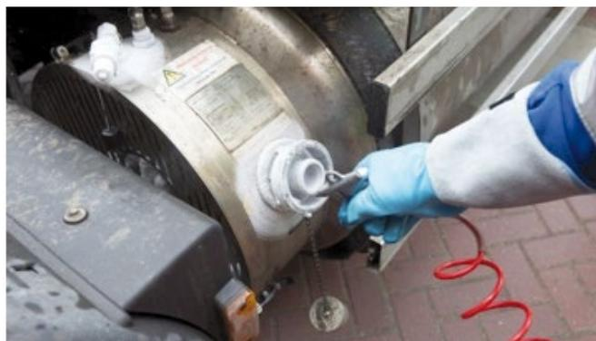
13 Unfasten the grounding cable and return it to the correct holder in the dispenser housing.
